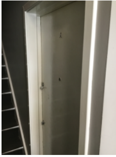
Typical flat entrance door.
