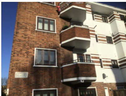
External walls front elevation.
