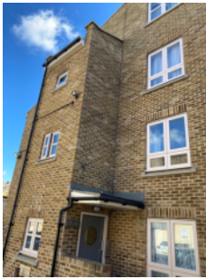
External walls - front elevation
