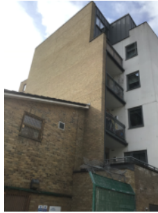
External walls on the eastern side elevation.
