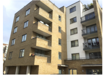
External walls on the western side elevation
