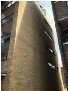
External walls on the rear (southern) elevation
