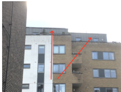
Photograph showing an identified external wall system on fifth floor
