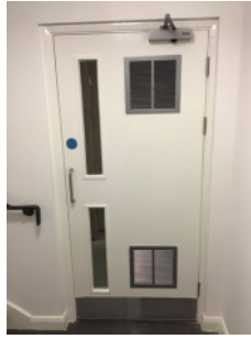
Grilles in basement doors
