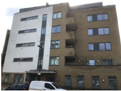
External walls on the front (northern) elevation
