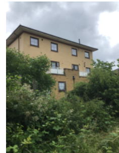
Rear elevation of building
