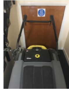
Confirm the electrical cupboard door is at least FD30S
