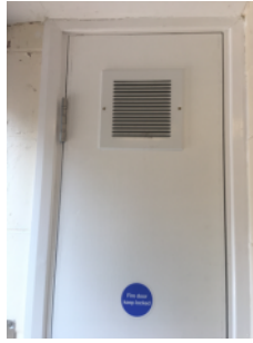
Vents in gas meter cupboard doors.
