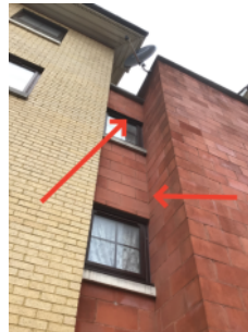
Central section appears to be vertical hung tile system
