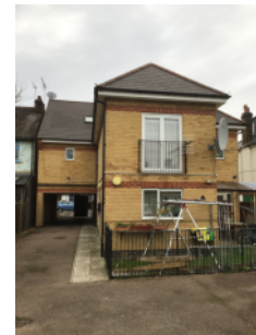
Brick/mortar external walls - rear elevation
