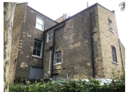
Brick and mortar external walls - rear elevation
