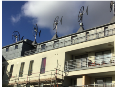
Unidentified wall cladding system on 4th floor
