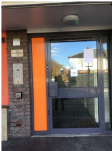
Firefighter override facility
