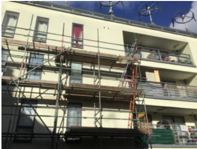
External wall - rear elevation
