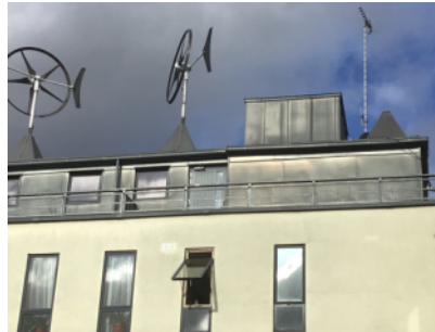
Cladding installed on 4th floor external walls
