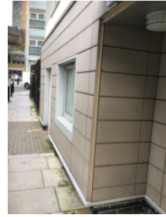
Tiles installed at ground floor level
