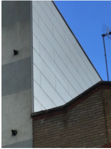
Unidentified wall system - 3rd and 4th floor, side elevation
