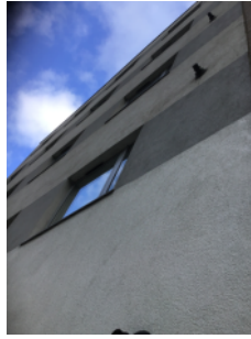
External walls rendered possibly directly applied on an insulating material
