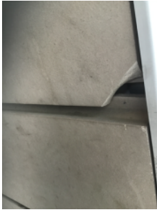
Concrete tiles installed on part of ground floor.
