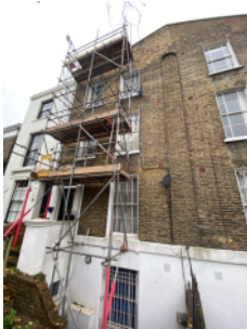
Scaffold erected on front face of building
