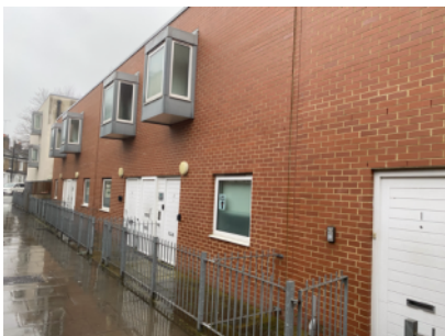
External walls – front elevation.
