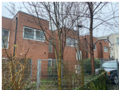
External walls – rear elevation.
