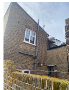
External walls - rear elevation
