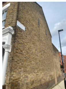
External walls - side elevation
