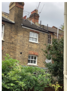
External walls - rear elevation
