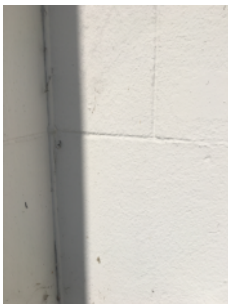
Close-up of render (mortar) applied to external walls
