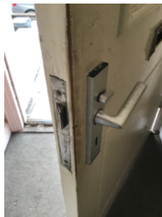
Mortice lock installed in main entrance door.
