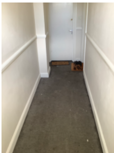
Entrance hallway found to be clear of obstructions and combustibles
