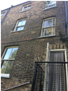
REAR ELEVATION: brick external wall
