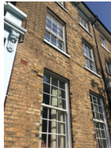
FRONT ELEVATION: brick construction.
