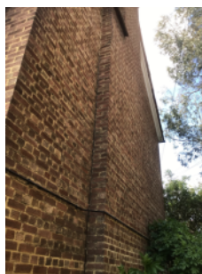
Brick/mortar construction, external walls, end elevation
