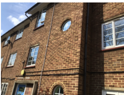
Brick/mortar construction, external walls, front elevation
