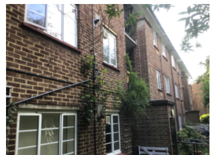
Brick/mortar construction, external walls, rear elevation
