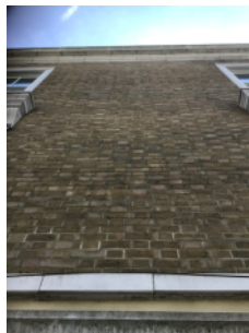
Brick/mortar external walls on 1st and 2nd floors
