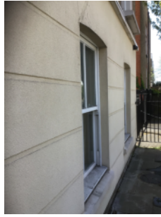
Rendered ground floor external walls.
