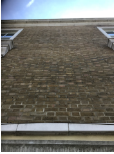
Brick/mortar construction of external walls.
