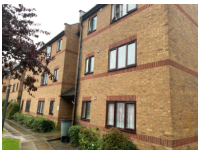
External walls - front elevation
