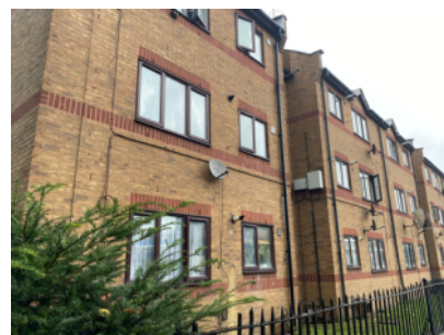
External walls - rear (roadside) elevation
