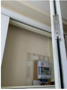
Strips and seals fitted on FD30S doors to electrical installations
