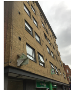
External walls, front of building
