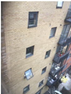
External Walls, rear of building.
