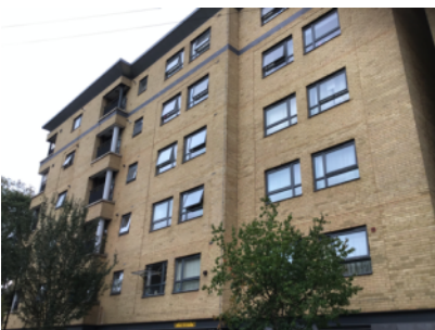
External walls, side face of building.
