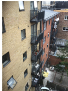
Steel protruding balconies at rear of building
