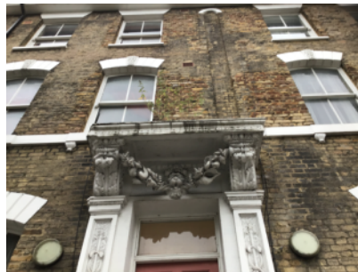
Front face - brick walls
