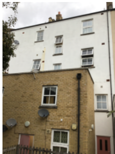
Rear face of the building - brick section, and a rendered section
