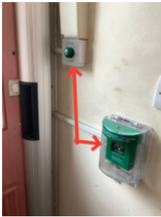
Electromagnetic door release, with additional emergency door release
