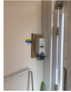
Should the fire alarm be removed, this meter should be in an FR30 enclosure
