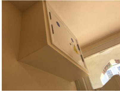
Photo showing electrical installations in an FR30 enclosure with FD30S door
