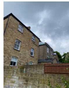
External walls - rear elevation
