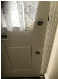
Thumb-turn devices fitted to main entrance door.
