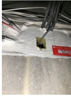
Cable penetration through installed fire stopping.
