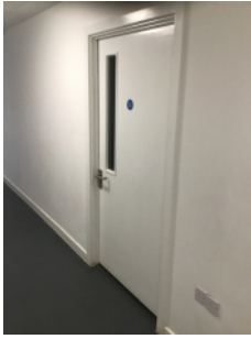
Access could not be gained into the pump room on the ground floor
