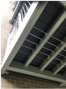
Timber decking provided as base for private balconies.
