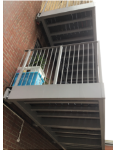
Private balcony construction
