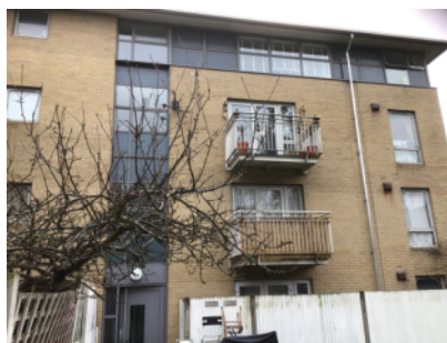
External walls – rear elevation.
