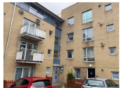
External walls - front elevation
