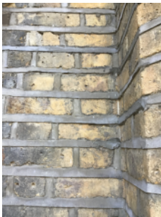
Original brick/mortar external walls
