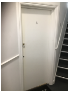
Example of FED in the building
