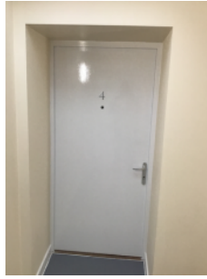
External condition of flat front door to flat 3.
