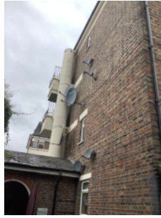
Brick/mortar external walls, end elevation.
