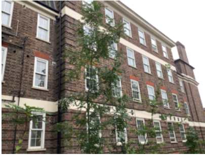
Brick/mortar external walls, end elevation.
