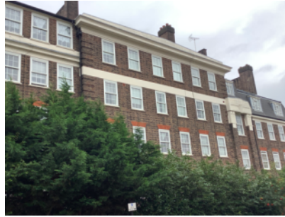
Brick/mortar external walls, rear elevation.
