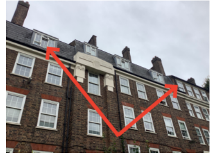
Vertically hung tiles, top floor
