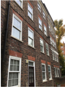
Brick/mortar external walls
