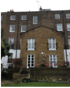
External walls – rear elevation
