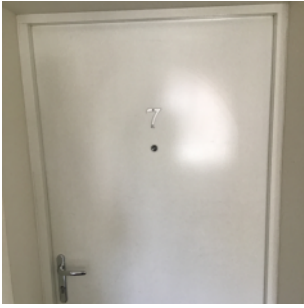
Flat entrance doors in good condition.
