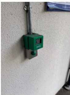
Electromagnetic gate release with emergency device.
