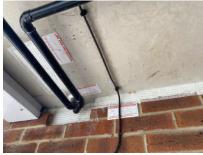
Fire stopping in the undercroft car park
