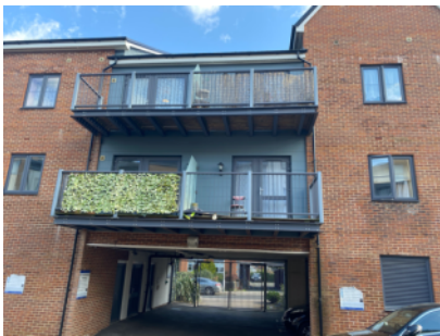
External walls, also showing balconies – rear elevation.
