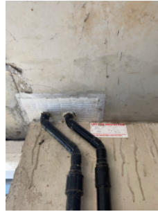
Fire stopping in the undercroft car park
