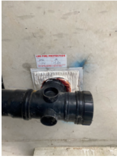
Fire stopping in the undercroft car park
