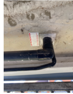
Fire stopping in the undercroft car park
