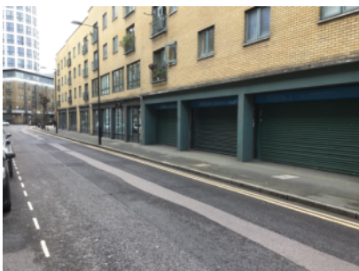
Commercial units occupy the ground floor of the building.
