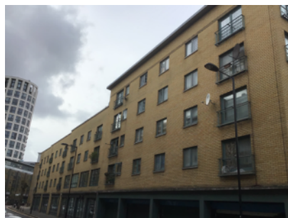
External walls (outside) of the building
