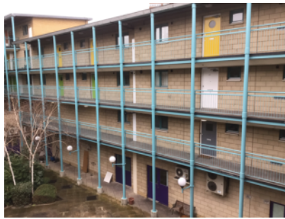
Windows and door glazing all above 1.1 m on common balconies.
