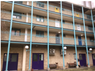
External walls (courtyard side) of the building
