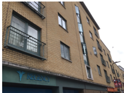
External walls (outside) of the building
