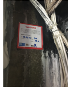
Evidence of fire stopping in riser cupboards
