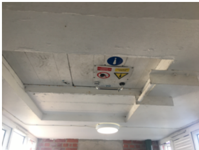
It was not possible to access the lift motor room
