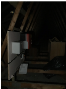
Photovoltaic solar power system in roofspace.
