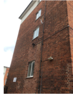
External walls, end elevation
