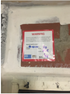
Evidence of recent fire stopping in riser cupboards
