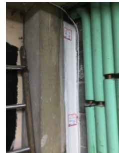
Fire stopping in the electrical cupboard
