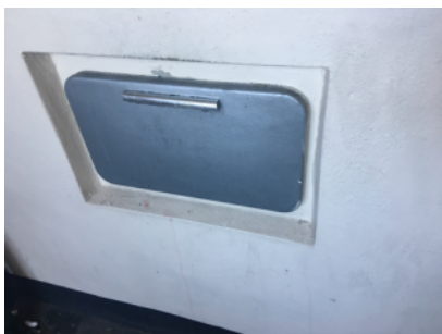
FR Flaps on rubbish chutes in good condition
