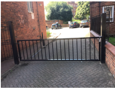
Entrance gate with fire service access key
