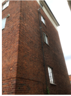
External walls, end elevation
