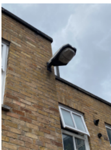
Street lighting immediately outside the building.
