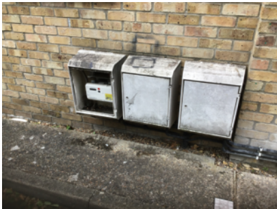
Gas meters located externally
