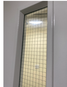
Georgian wired glazing in lobby doors
