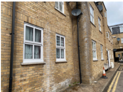
External walls - front elevation
