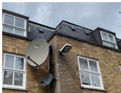
Street lighting immediately outside the building.
