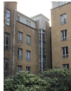
External walls-rear elevation.
