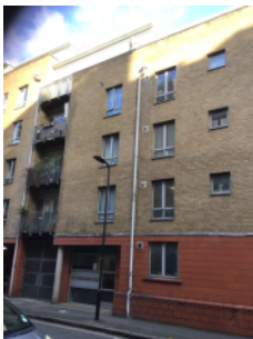
External walls - front elevation
