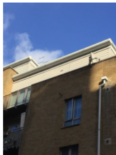
Unidentified EWS fitted on the fourth and fifth floor
