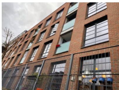
External walls – Rear elevation.
