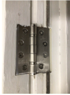
Door hinges to BS1935 and CE1121 on FD60S riser doors
