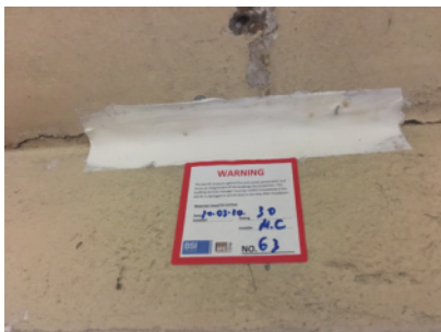
Evidence of recent fire stopping
