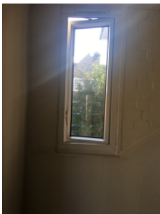
Openable windows in staircase
