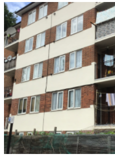
External walls, rear elevation
