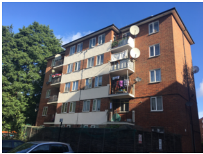
Residents have private balconies at the rear of the building.
