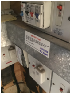
Evidence of EIC testing
