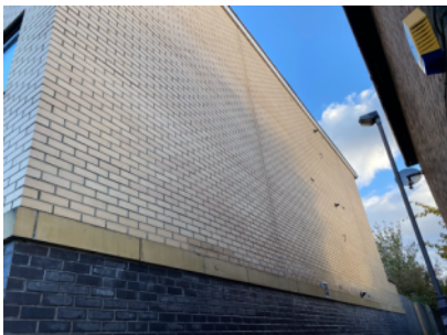
Brick/mortar faced external wall - side elevation
