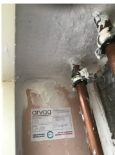
Fire stopping installed in October 2019
