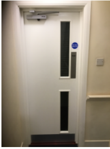
Example of lobby doors fitted in the building
