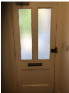
Secured main entrance door can be unlocked without need of a key
