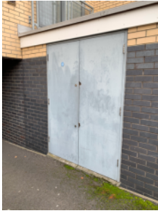
It was not possible to access this external door.
