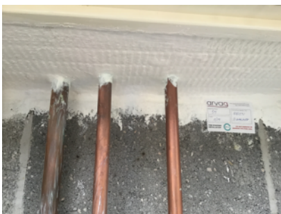
Evidence of recent fire stopping.
