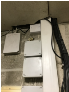
Cable penetrations in the ceiling of the electrical cupboard
