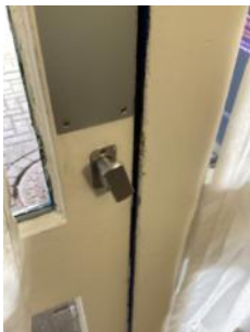
Front entrance thumb turn device.
