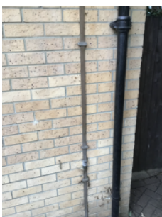
Lightning conductor
