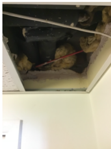
Possible penetrations between common area and flat above false ceiling
