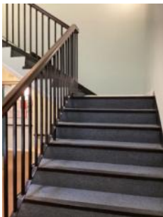
Escape route with contrasting stair nosings
