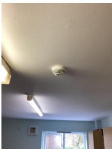
Heat detector in common kitchen
