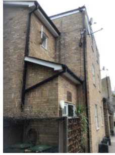
Brick/mortar external walls- front elevation
