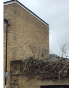
Brick/mortar external walls- side elevation
