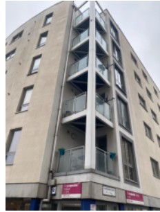
Private balconies, steel framed, steel deck, glazed up stands.
