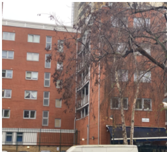
Rear elevation also showing common balconies.
