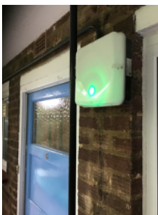
Non-maintained emergency lighting provided on common balconies.
