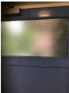
Georgian wired fanlights in staircase doors.
