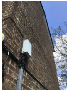
External walls – end elevation
