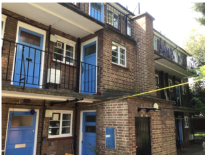
External walls – rear elevation
