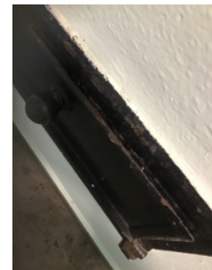
Refuse chute located in the staircase.
