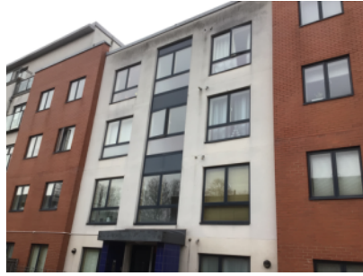
External walls - front elevation
