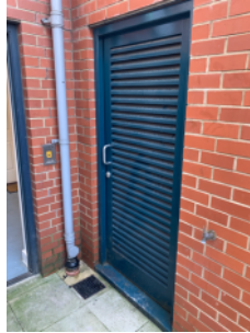
Access was not possible into this door.
