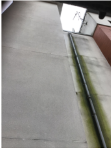
External walls – rear elevation
