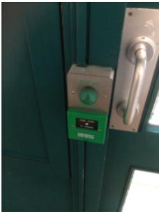
Electromagnetic door release with emergency override is provided
