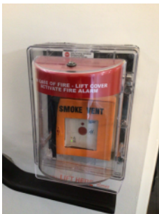
Incorrect signage on AOV control
