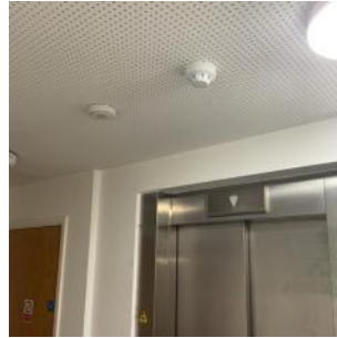
Smoke detection in lobby to operate smoke vent
