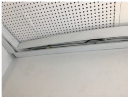
Showing cables within plastic ducting affixed to the ceiling in common area
