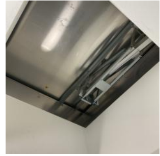
AOV in staircase manual smoke vent
