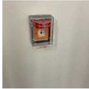
Manual smoke vent control
