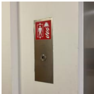
Firefighter lift override facility
