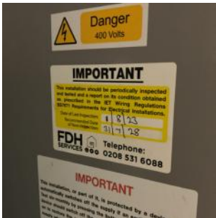
Fixed wire test in date
