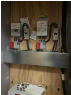
Electric meters in riser cupboard
