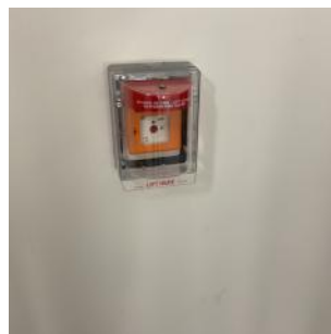
Manual smoke vent control
