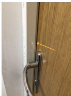
Possible surface mounted smoke seal
