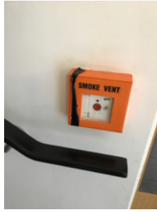
Smoke Vent controls held shut with tape
