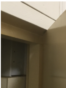
25mm door stops on electrical cupboard.
