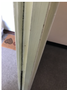
Missing section of smoke seal
