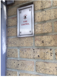
Defective override facility
